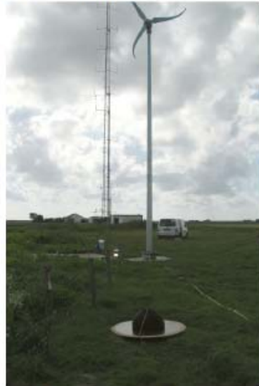
Photo1: Picture taken from the board in toward the WTGS
